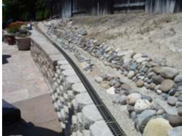
The backyard with the stone-lined stream bed. This view shows two kinds of dry-laid concrete blocks which make an excellent low retaining wall.
